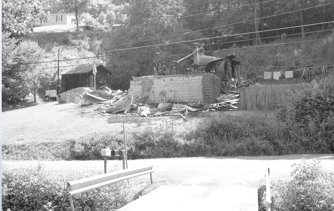
The burnt remains of Nick Mullins' great-grandparents' home place that Nick was remodeling. The cause of the fire was electrical.
