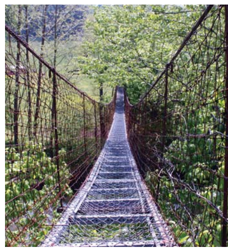
Swinging bridge in Clay County.
