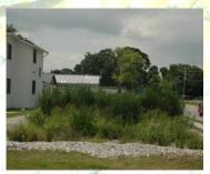
The subsurface wetlands receive water from the Ecological Machine biological wastewater treatment greenhouse, and provide further improvement in water quality. Because the water level remains below the gravel surface, there is no possibility of mosquito larvae breeding or child hazards. Water from the wetlands passes through an ultraviolet sterilizer and then returns to the Ecovillage apartments for use in flushing toilets. This saves up to 350 gallons per day of municipal water.
