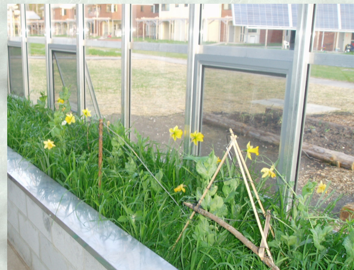
The greywater treatment system cleans water from bathroom sinks and showers.
