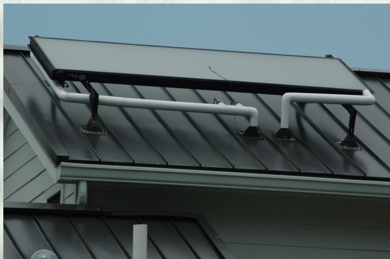
A SunEarth Imperial Flat Plate Collector uses sunlight to heat water for the house.
