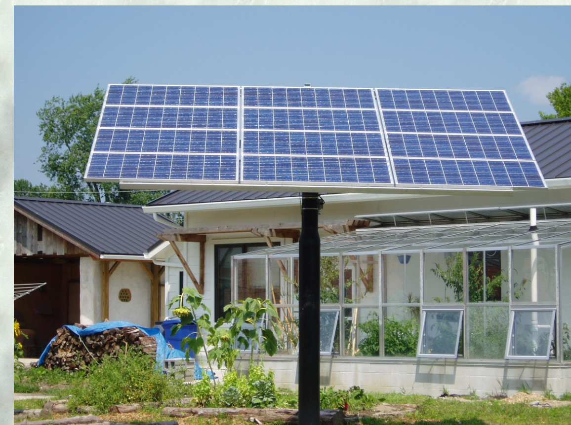
A 1500-watt photovoltaic array tracks the sun as it converts sunlight into electricity.
