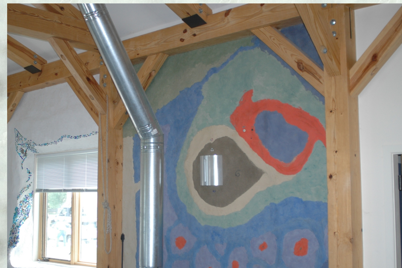
Post-and-beam construction frames a straw bale wall.
