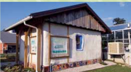
Straw Bale Construction at the Information Kiosk
