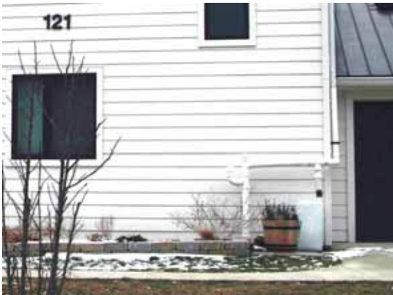
Downspouts Collect Rainwater for Reuse
